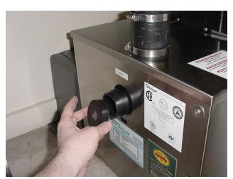
Before Installing the HAG Horizontal Air Gap Assembly, remove the Flow Control located on the Inlet end.
