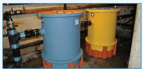
A Solids Separator installed ahead of a Trapzilla® GI for the food prep area of a national grocery chain.
