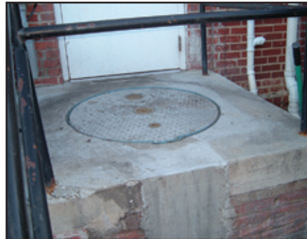
TZ-600 Installed in Stairway Landing behind Restaurant
