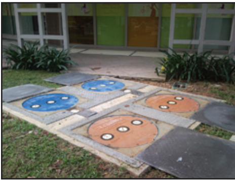
Two TSS-95 Solids Separators in front of two TZ-600 Grease Interceptors servicing a large cafeteria in a high-rise office building.
