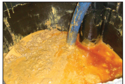
Grease being removed from TZ-600 in International Fast Food Chain.
