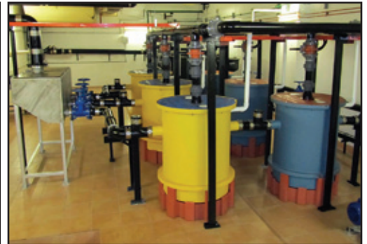
Trapzilla® Grease Interceptors and Solids Separators Servicing a Major International Hospital
