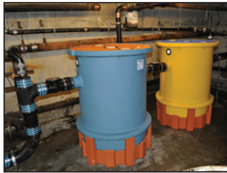
A Solids Separator installed ahead of a Trappzilla® GI servicing the food prep area of a national grocery chain.
